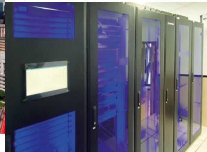
Energy-efficient solution: Mini Data Centre with integrated in-row cooler
