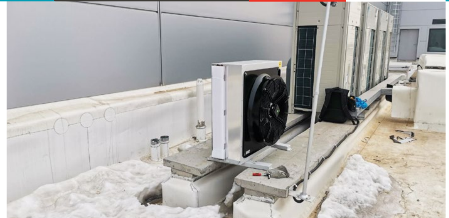
Installing the air conditioning unit for the Mini Data Centre
