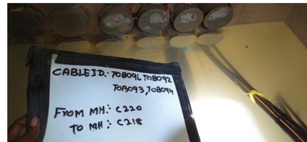
Cable run-in in ducts which are periodically filled with sea water
