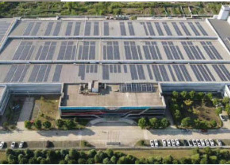
Greenelectricity from the roof of the factory in China.
