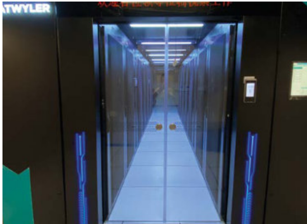
Installation and commissioning of the equipment was completed within a week.
