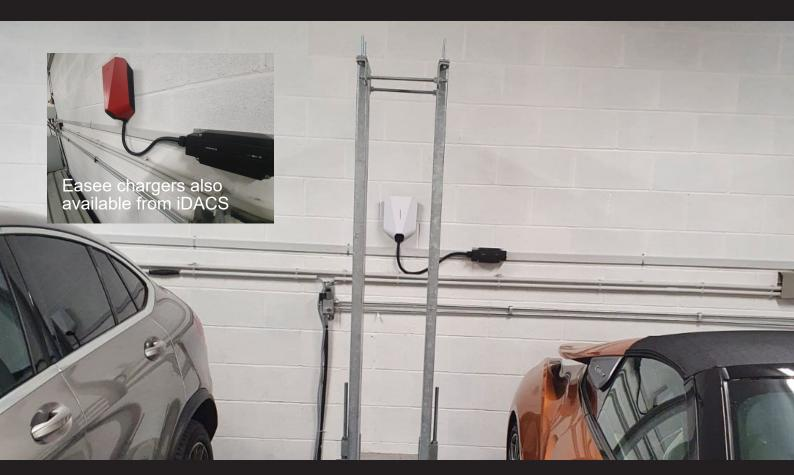
Flexible and extendable infrastructure for your parking. The Woertz flat cable system allows you to install the infrastructure first and add chargers as your need for charging stations grows.
