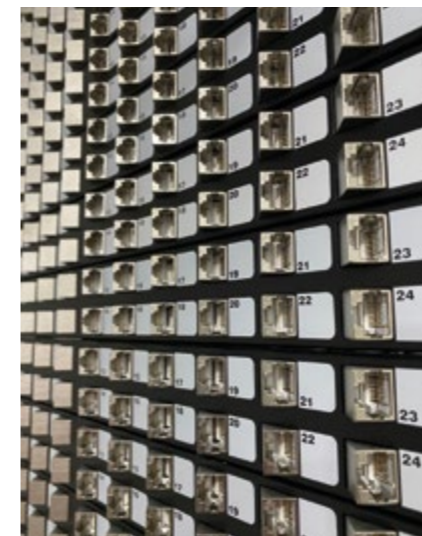
Patch panels with angled RJ45 modules
